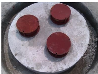
(c) 刚度调节装置安装
